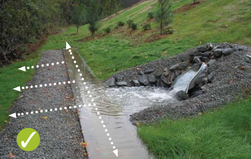
Good application of level spreader at outfall from large ponding basin. Flows plunge into small pool, spread out evenly across level concrete lip, then sheet flow from lip across gravel into grass (Source: NC State University).
