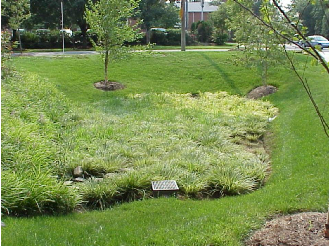
Figure 5.9 Typical Application of a Bioretention Filter
