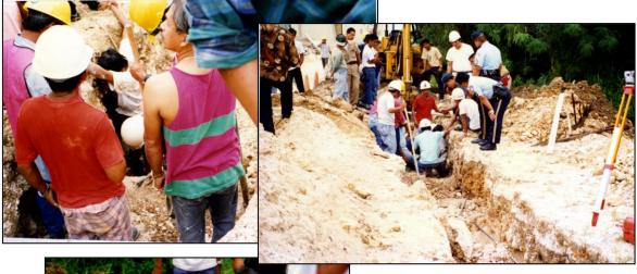
Figure 4.1: An actual trench collapse accident in the Lower Base area of Saipan. The depth of the trench was about 5 feet. Soil type appears to be either backfill, or coastal alluvial sediments, which are very common along Saipan's west coast. Note the severely broken leg.
